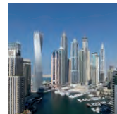
DUBAI Saving energy in air conditioning systems
